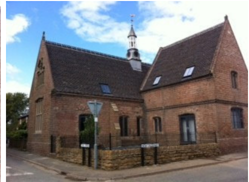
Refurbished complete with clock tower!
