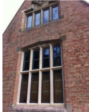
New windows and refurbished stone surrounds
